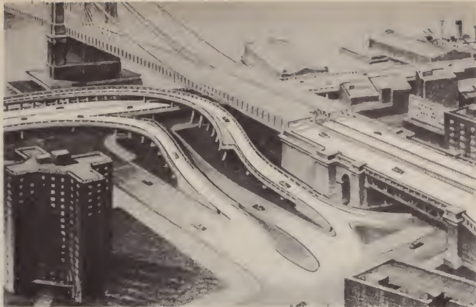
Construction of on and off-access ramps from the South Street Elevated Highway — bringing traffic to grade at Pearl Street, is expected to be undertaken in the coming year.
